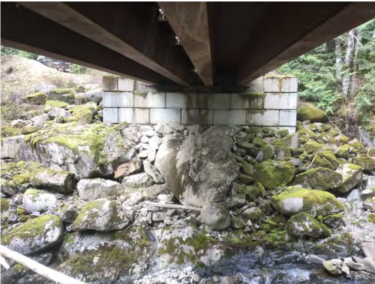
Right Bank Abutment when facing downstream
