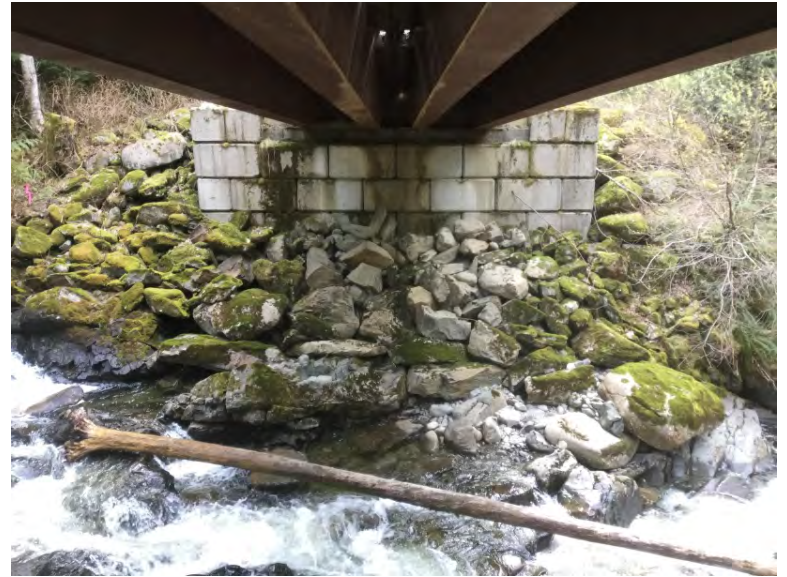
Left Bank Abutment when facing downstream
